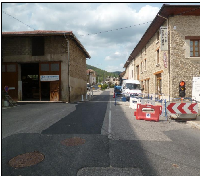
Travaux centre village
